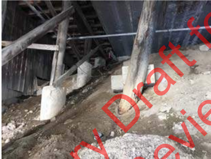
View of the southern culvert under bridge/restaurant.
