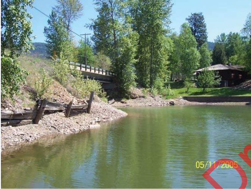
Shoreline Type 8C: Sheltered riprap
