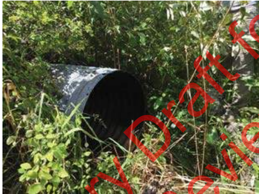
14 inch culvert South of railroad trestle.
