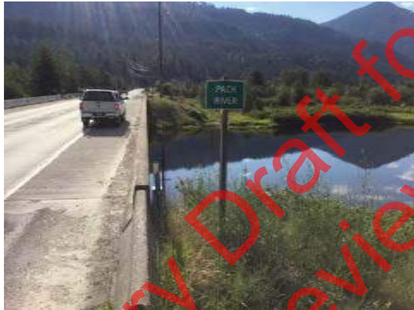
Pack River bridge from SR200 east bound.
