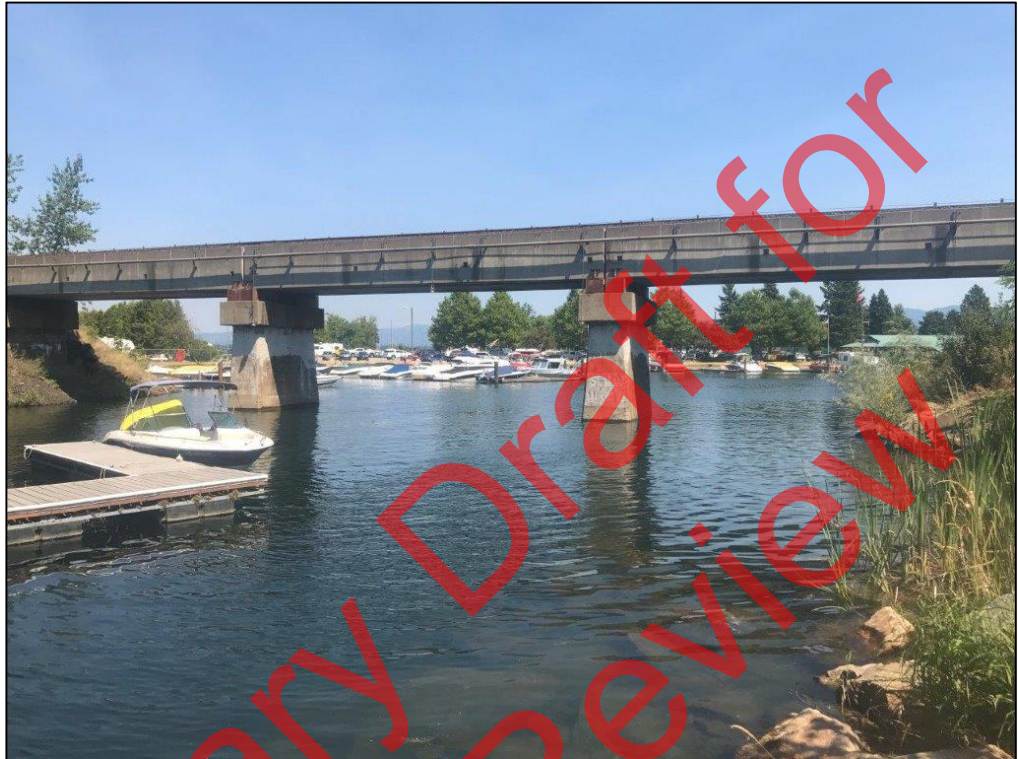
Figure 7. The Sandpoint Marina dock within BNSF ROW, upstream of the existing Br 3.1
