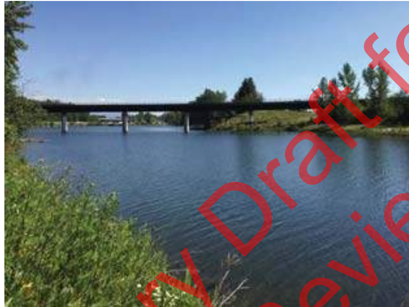
Looking north from River right towards the trestle.
