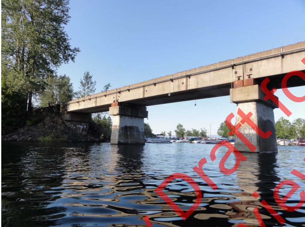
Key View 2a: Bridge 3.1 over Sand Creek, viewing northwest from the water.
